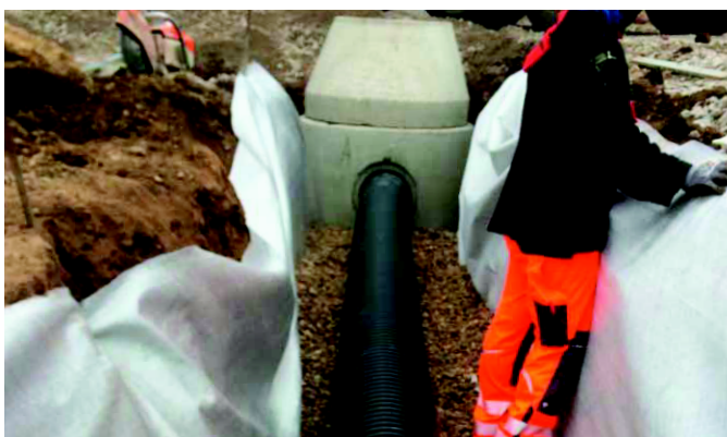
Drainagerohr in Schotter
